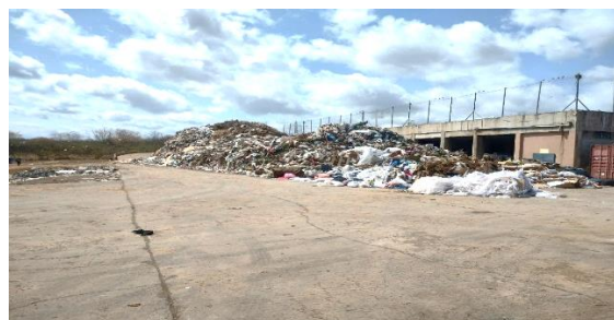
Figure 10 Near Concrete Platform
