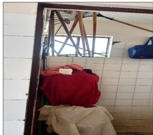
Figure 8 Cleaning Materials Stored inside toilet block
