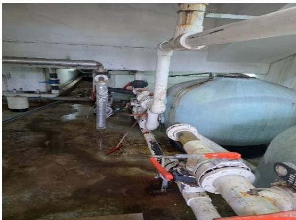
Figure 11 Condition of Plant room
