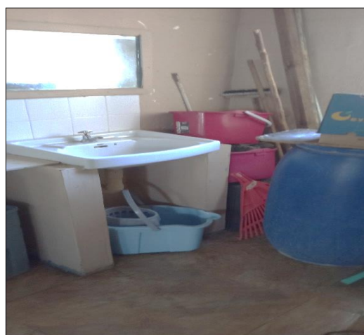
Figure 4 Cleaning Materials stored inside toilets
