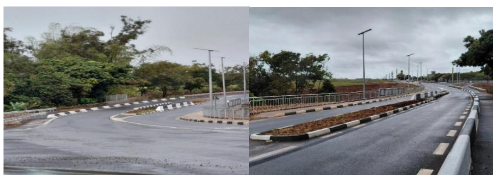
Figure 7 Construction of new Bridge and Road Alignment at Riviere Dragon
